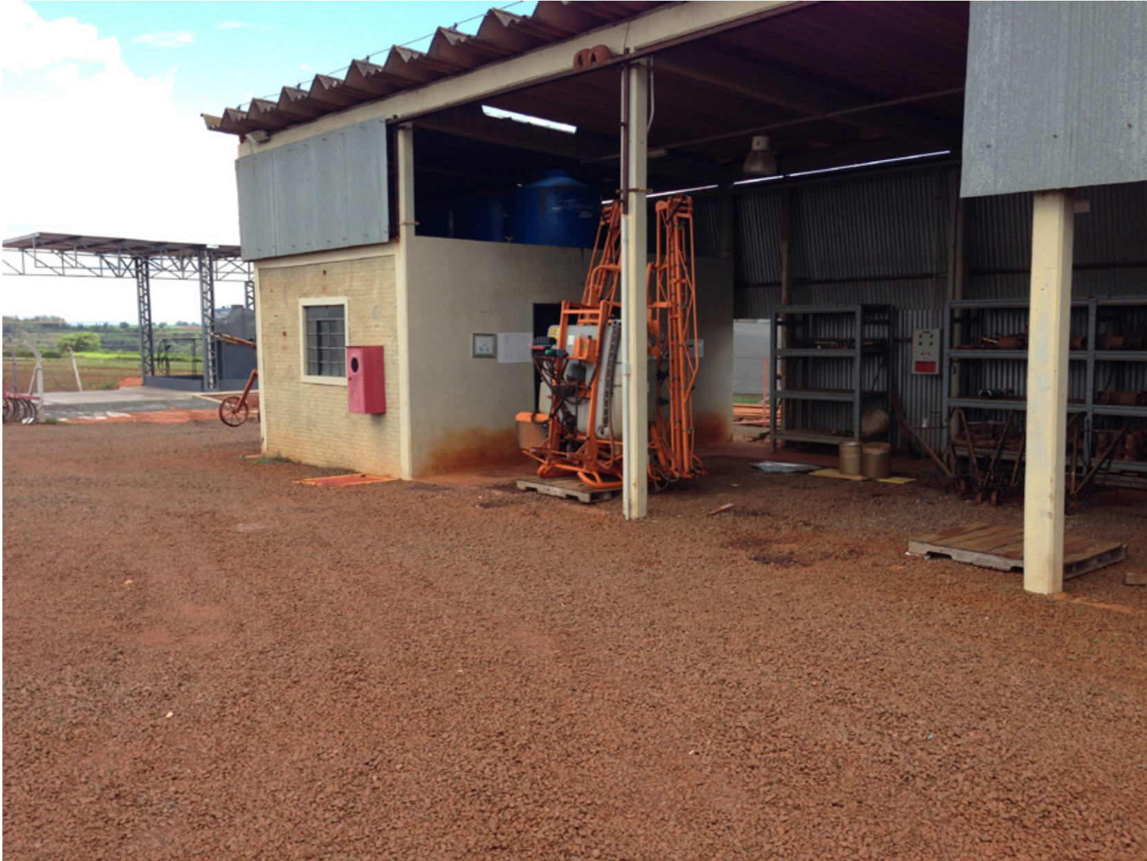
Fire Protection Device
