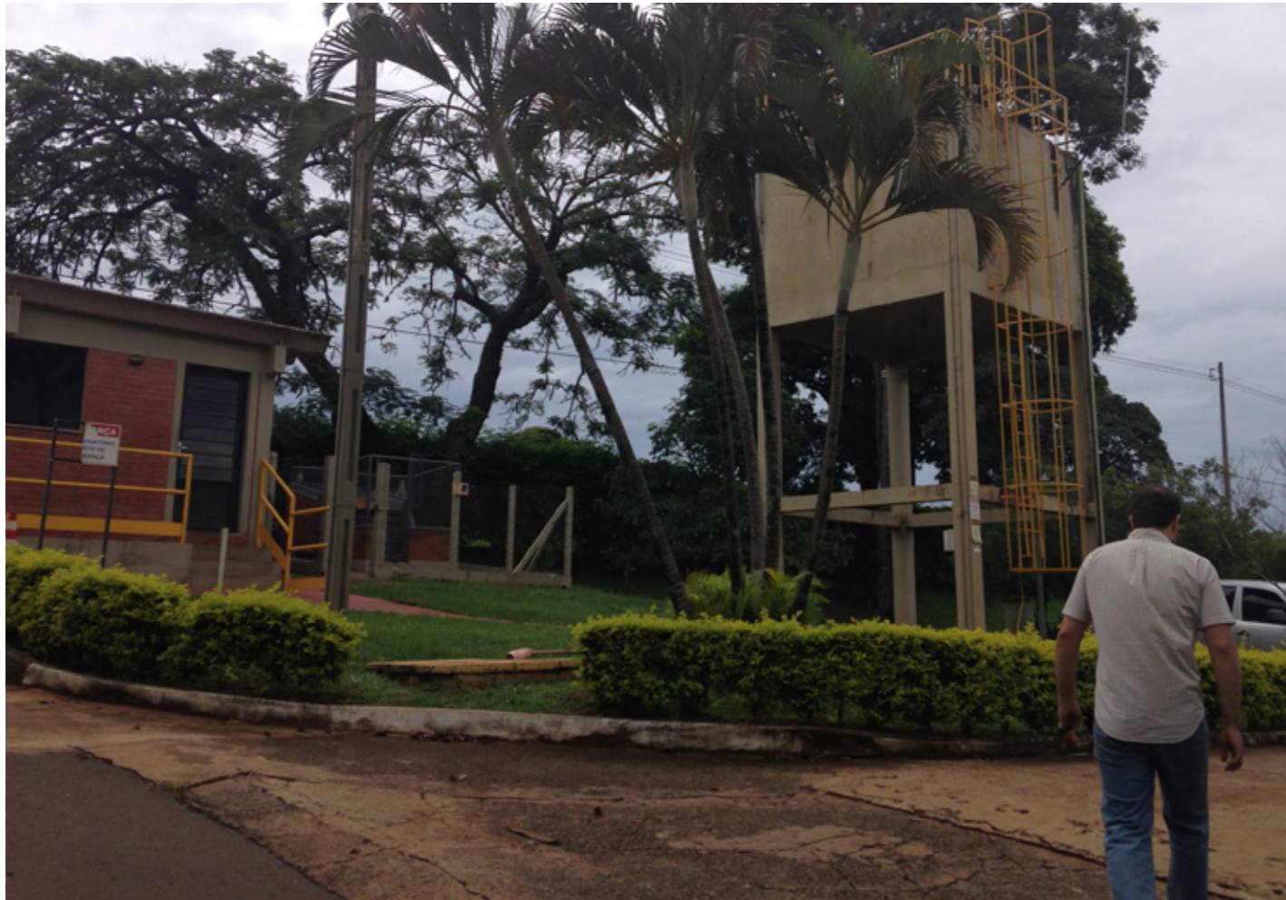
Water tank to be deactivated (#3)
