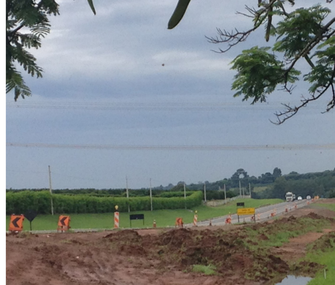
Highway Duplication Works
