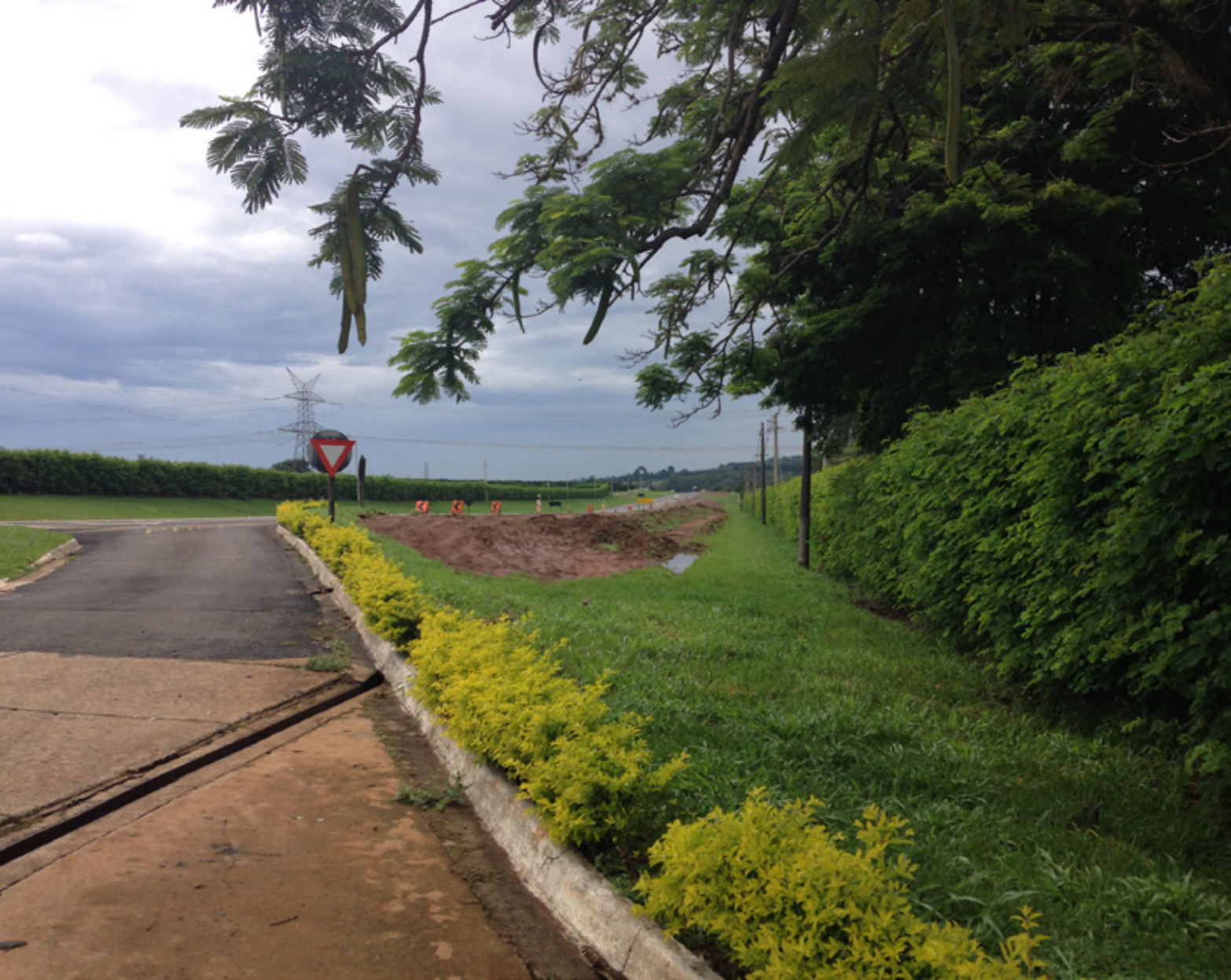
SP-147 Highway Duplication Works
