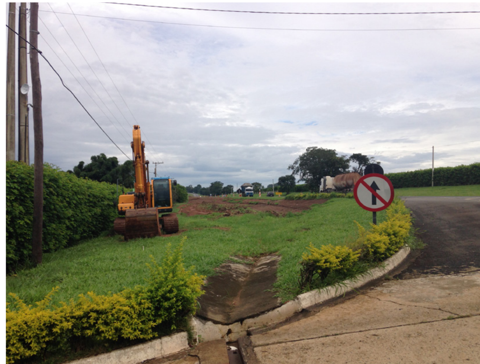
SP-147 Highway Duplication Works
