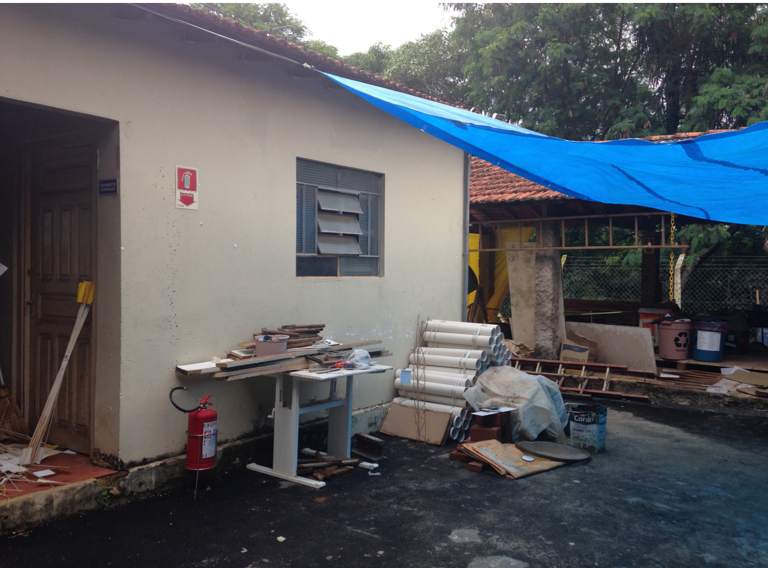
Storage building to be demolished
