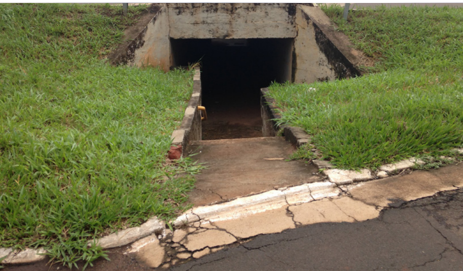
Pedestrians underground passageway - South
