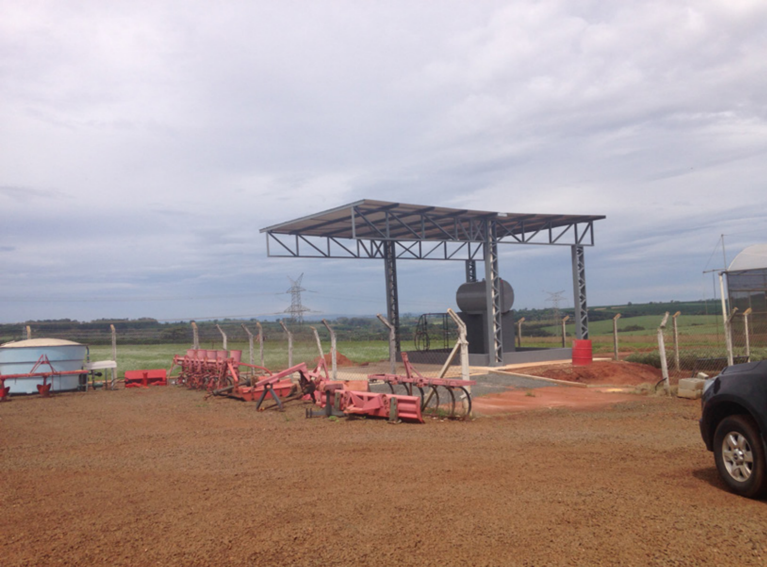
Fuel Station - North Site (#30)
